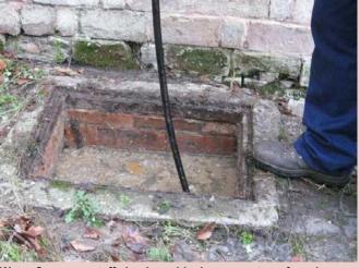
Water Company staff clearing a blockage on a transferred sewer
